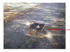
Pavement repair needed:
