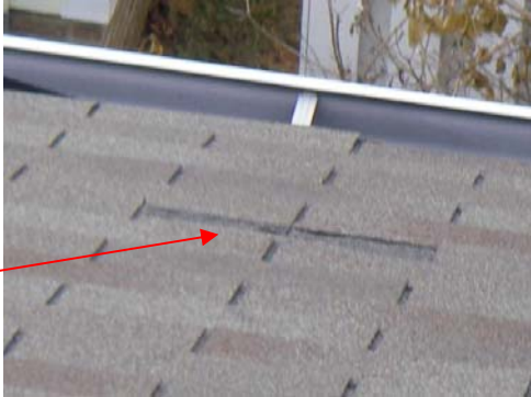
Sample – roof repairs: Loose shingle Missing shingle
